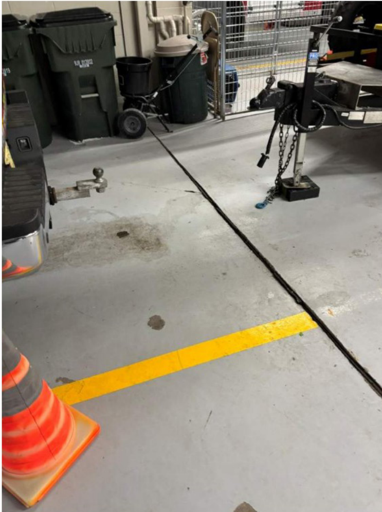
Photo 16: Transition at original floor (ground supported floor) to precast plank floor – The ground supported floor has settled due to lateral movement of the basement walls below. The floor should be leveled using foam injection, then properly sealed and coated to prevent moisture intrusion.
