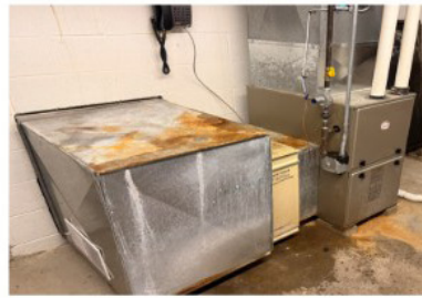
Payne HVAC Unit – Basement Area
