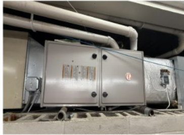
Payne HVAC Unit – 1 st floor Office Area
