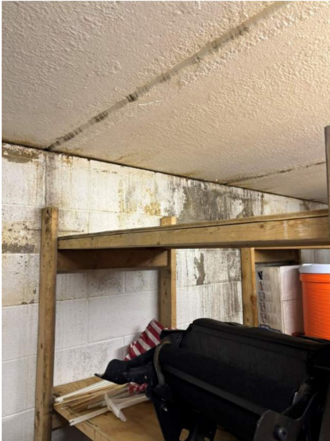
Photo 19: South Exterior wall. Evidence of water infiltration from the floor above and from outside water sources.
