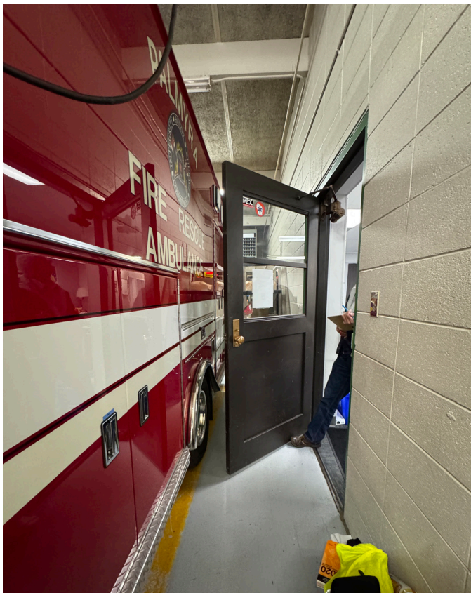
NON-CODE COMPLIANT EXIT AND UNSAFE PATH OF RESPONSE TRAVEL
