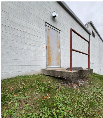
RUST ON DOOR AT NORTHEAST WALL
