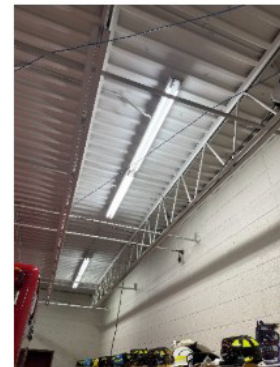
Data wiring not properly supported
