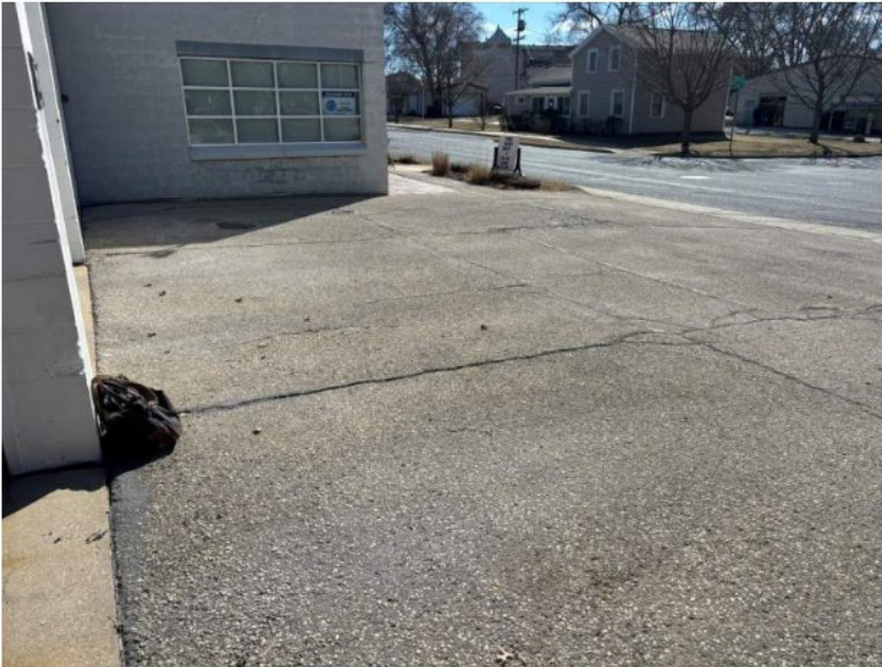
Photo 15: Exterior pavements are in poor condition.
