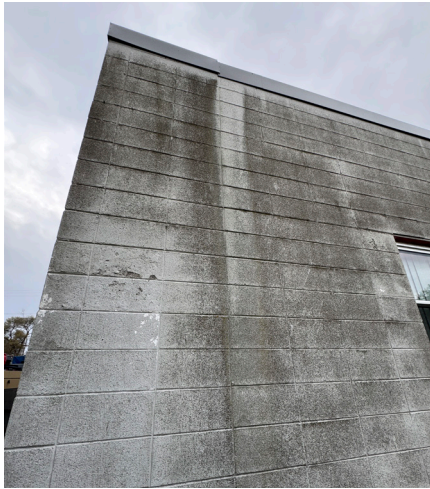
NORTHEAST WALL CONDITION FROM WATER RUNOFF
