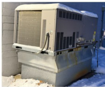
Carrier WeatherMaker® packaged rooftop gas heat and electric cool unit – ground mounted
