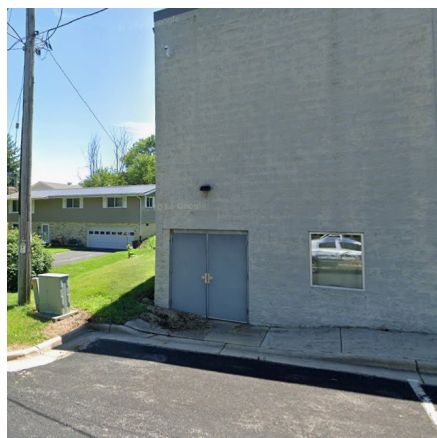
SITE EROSION AT BASEMENT DOORS
