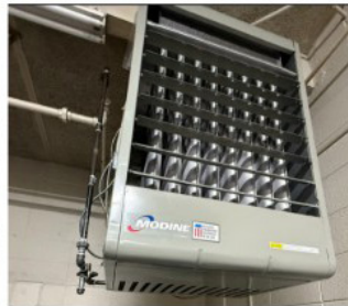
Unit Heater – HVU2 – Middle Bay
