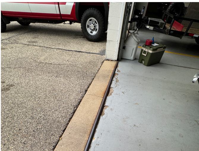
DAMAGED SLAB EDGE & LIKELY LOCATION FOR WATER INFILTRATION INTO BASEMENT
