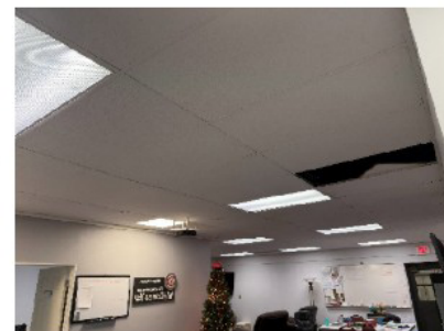
Typical Light Fixture
