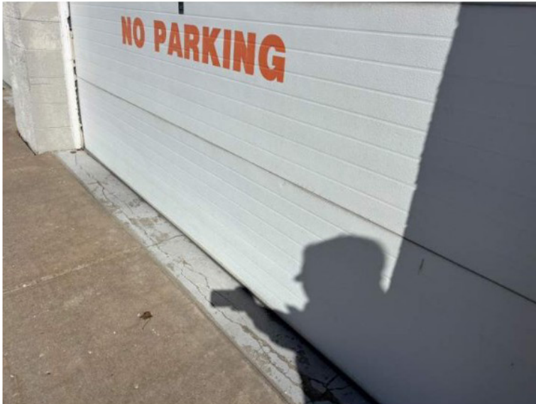
Photo 9: South Apparatus Bay doors – close-up view of threshold – damaged topping allows water to penetrate. Topping should be repaired / replaced and coated to prevent moisture intrusion.
