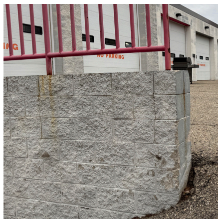
RETAINING WALL CRACKING
