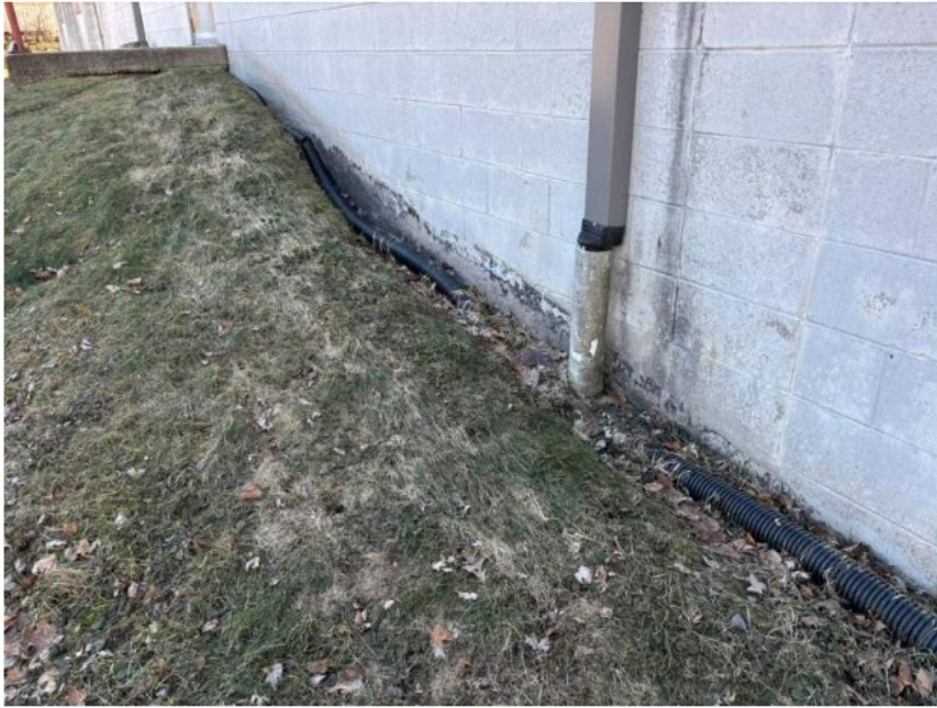
Photo 24: North exterior wall, note inadequate drainage, waterproofing system appears deteriorated, surface water would be directed to the wall surface.
