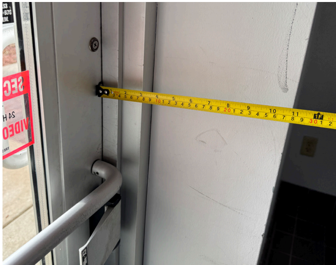
NON-ADA COMPLIANT EXIT DOOR
