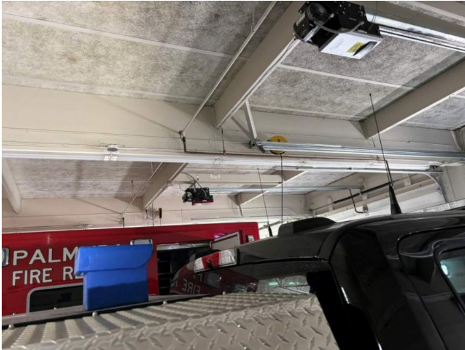
Photo 12: Original roof structure – timber with gypsum panel decking, appears to be performing adequately.
