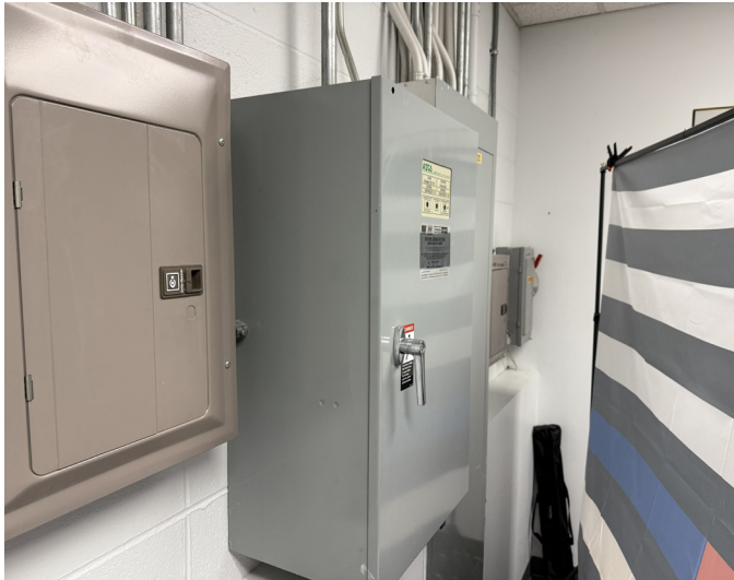
POLICE CHIEF OFFICE WALL LINED WITH ELECTRICAL PANELS
