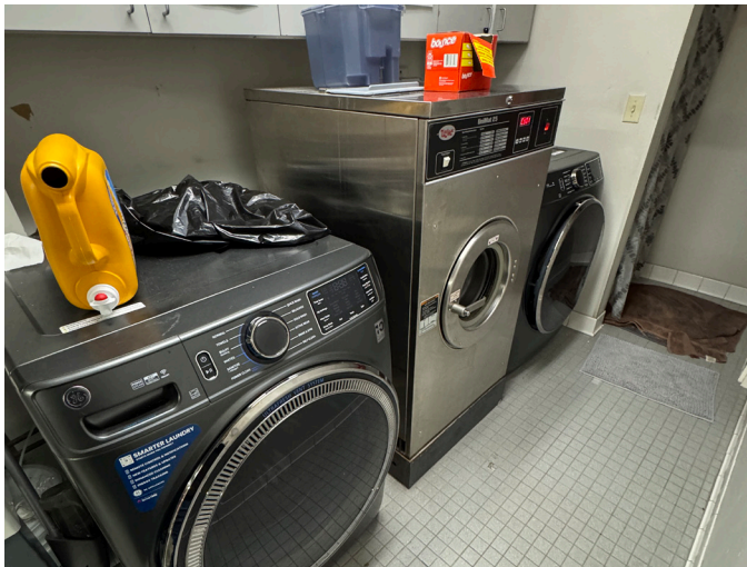
SMALL DECON ROOM WITH NON-ADA COMPLIANT SHOWER
