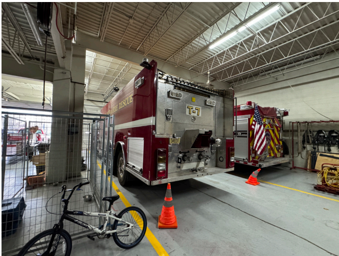
INADEQUATE LIGHTING LEVELS IN APP BAY
