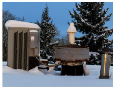
Rooftop Condenser & vents
