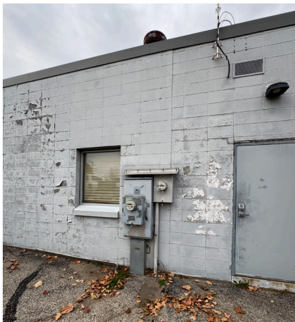
SOUTHEAST WALL PAINT PEELING OFF CMU
