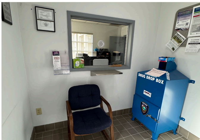
MAIN ENTRY VESTIBULE NON-ADA COMPLIANT TRANSACTION WINDOW
