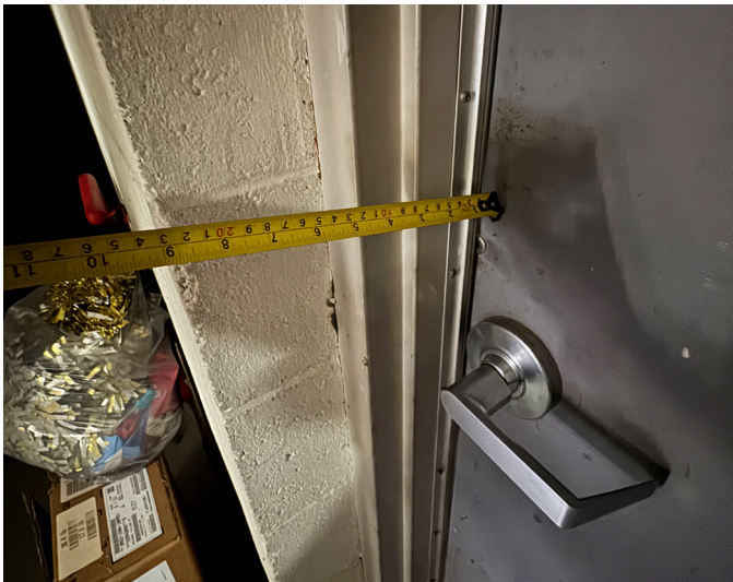
NON-ADA COMPLIANT EXIT DOOR
