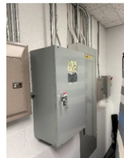
ATS and Main Panel
