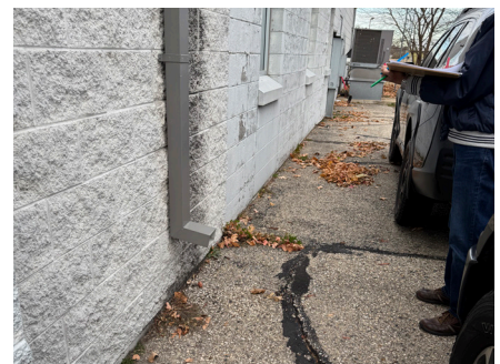
DOWNSPOUT DRAINS AT GRADE AT PARKING
