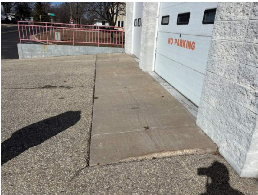
Photo 8: South exterior wall o pavements are in poor condition, transition concrete toppings at the overhead doors are cracked and should be replaced and coated with a traffic coating to prevent water intrusion. Waterproofing along this wall appears to also be inadequate (see basement photos)
