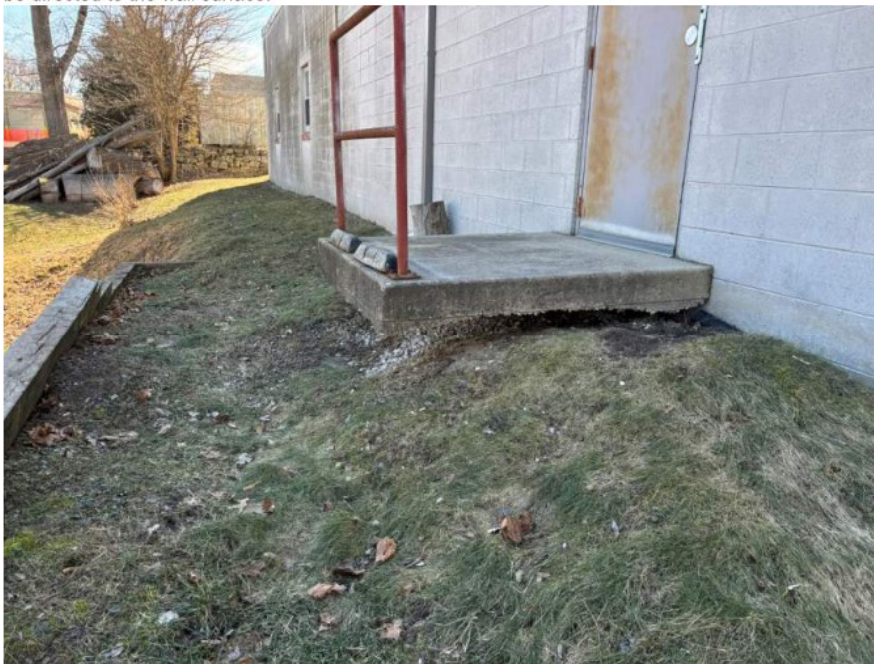
Photo 25: Stoop slab is not supported and therefore not safe as an exit. It should be closed off, until it can be repaired or replaced.
