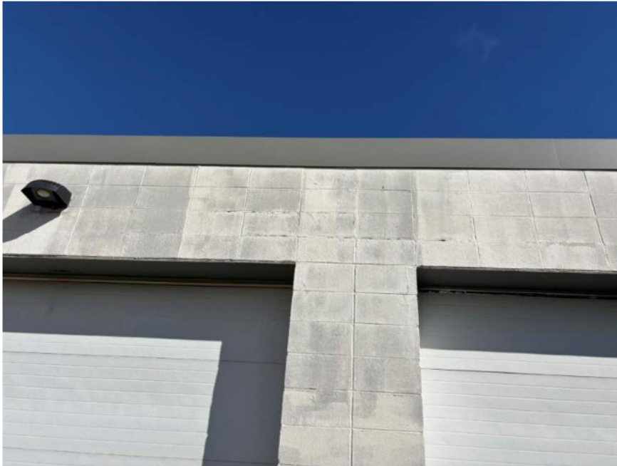
Photo 7: Exterior wall coatings are in poor condition.
