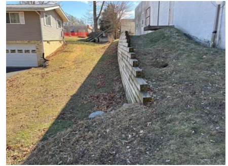
WOOD RETAINING WALL AND ADJACENT SITE EROSION
