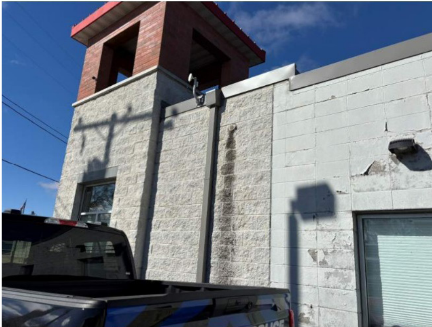
Photo 5: East exterior wall looking southwest – note deteriorated masonry coatings, exhaust vent should extend further out etc. to protect the integrity of the masonry walls.
