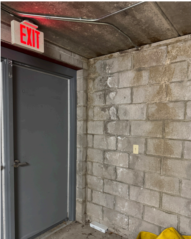
EVIDENCE OF WATER INFILTRATION AT BASEMENT WALLS
