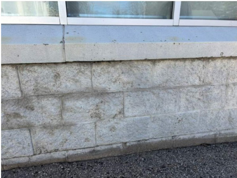
Photo 6: Caulk Joints on the Sills are in poor condition, allowing moisture into the wall, which if not corrected, will deteriorate the masonry walls.
