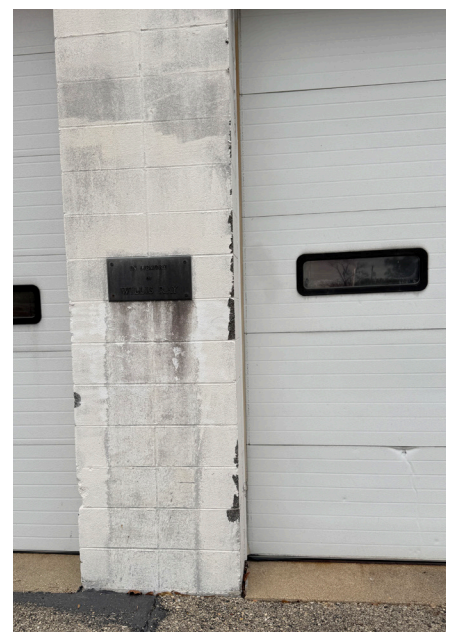
DAMAGE TO OVERHEAD DOOR JAMBS
