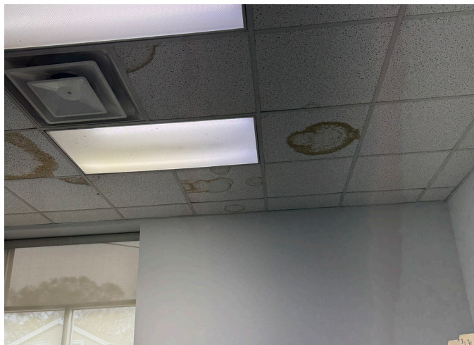
POLICE DISPATCH DAMAGED CEILING TILES
