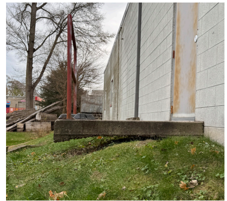
UNDERMINED EXIT STOOP
