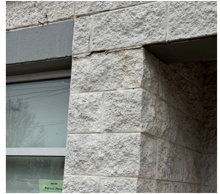
CRACKING & SEALANT FAILURES AT ENTRY
