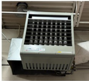
Unit Heater – HVU1 – Left Bay
