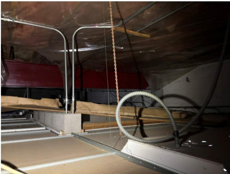
Photo 13: Roof structure above the meeting room space.
