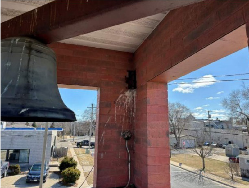
Photo 14: Bell Tower Structure at SE corner of the building. Note a large hole in the masonry should be repaired to prevent water infiltration.
