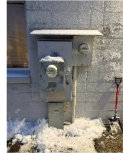
Meter on Exterior Wall
