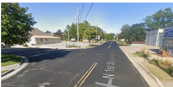
LOOKING NORTHWEST ON N 1ST ST. - NO SIGNS, OR MARKINGS WARNING OF RESPONSE TRAFFIC
