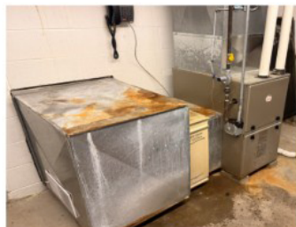
Payne HVAC Unit – Basement Area
