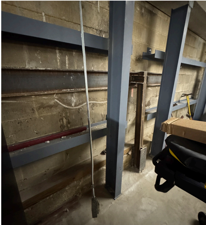
TWO PREVIOUS STRUCTURAL REPAIRS ALONG BASEMENT WALLS
