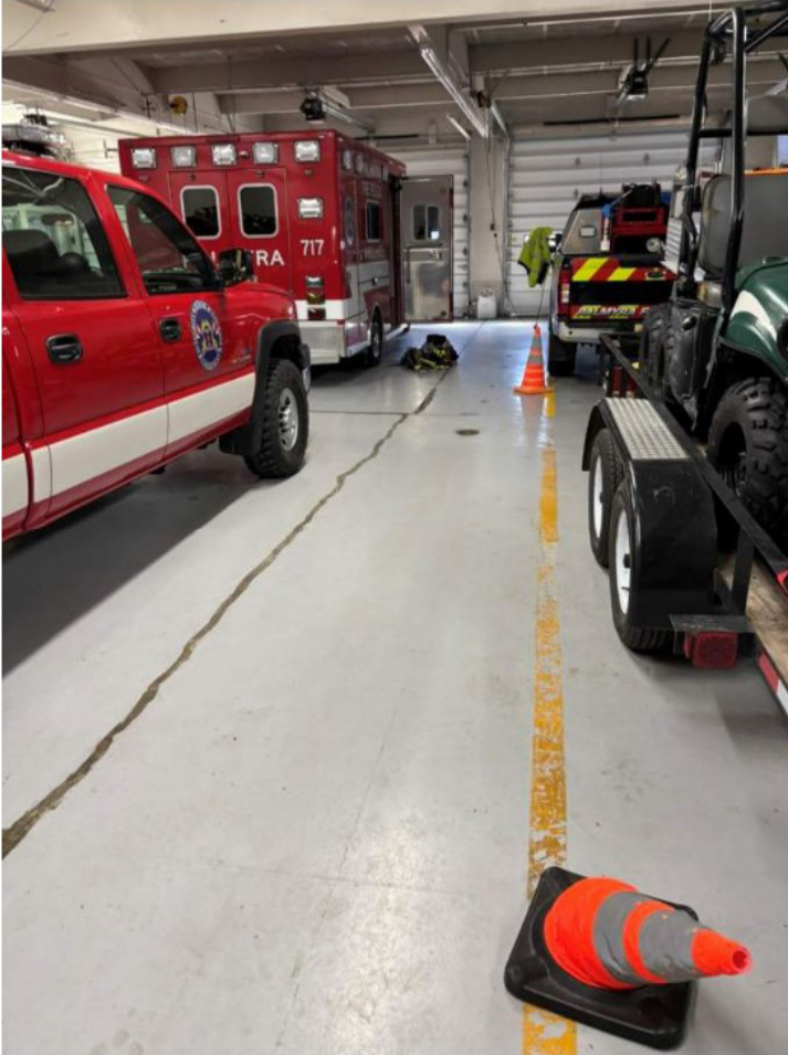
Photo 11: Interior of 1997 Apparatus Bay – Note cracks have been sealed, however the users report that they do not wash in the bays due to excessive leaks. The floor should properly coated with a traffic coating / waterproofing to protect the floor plank. Note vehicles parked in the bays are not excessively heavy, but we did not observe signage for guidance on maximum axle loads.
