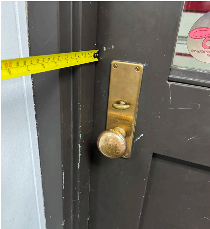
NON-ADA COMPLIANT EXIT DOOR
