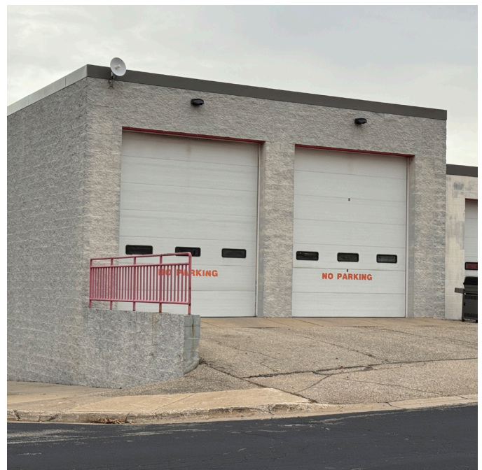
RETAINING WALL AND STEEP SLOPE AT APPARATUS BAY APRON
